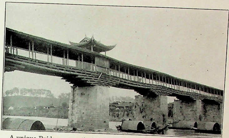
A unique Bridge across the River at Kienyang, North-west Fukien.
