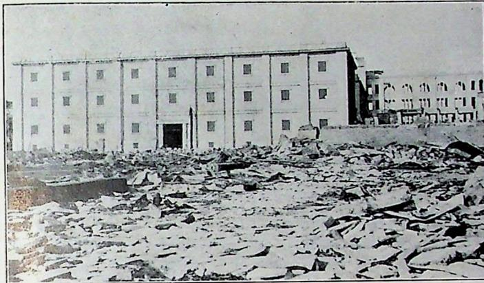
The only building intact in Yokohama. Reinforced concrete structure designed by American architects.
