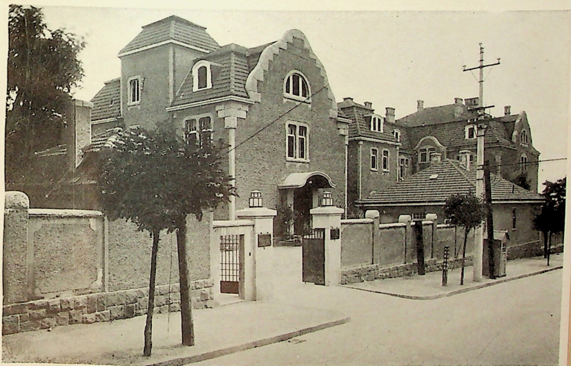
Above, the Isolation Ward and, below, the main Building of the Faberkrankenhaus in Tsingtao. This German-run Convalescent Hospital was first opened in 1907, and is largely patronized by the Foreigners residing on the Shantung Peninsula.
