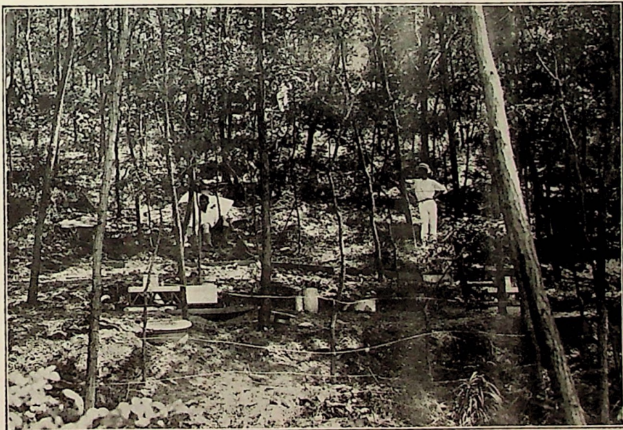
Experimenting on Surface Run-off of Rainfall at Tsingtao. This is the Plot chosen in the Area planted by the Germans. An enormous difference was noted between the Run-off from this Plot and that from a denuded Plot in the neighbouring Hills, the Run-off from the latter being almost fifty times as great as that from the former. The extreme importance of Slope Reclamation by Afforestation is amply demonstrated by these Experiments.
