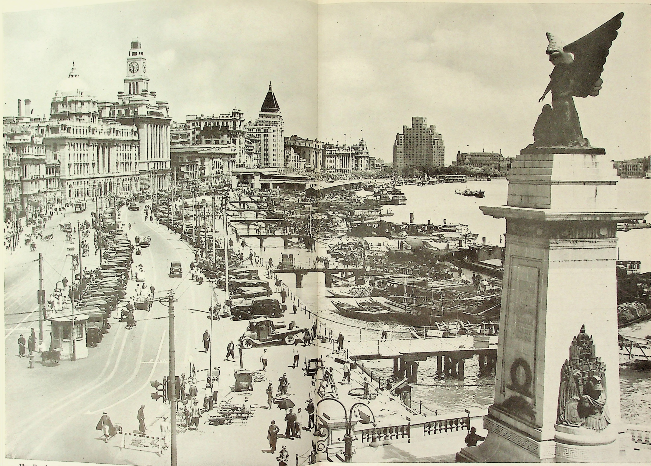
The Bund and magnificent Water-front Buildings of Shanghai to-day, the Four largest being the Hongkong and Shanghai Bank, the Customs Building, the Cathay Hotel and the Broadway Mansions. In the Right foreground is the Cenotaph. This beautiful Picture was made by Eastman Kodak Company, Shanghai.
