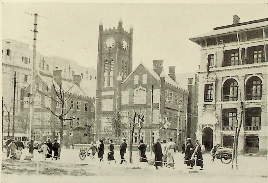
The Customs Building on the same Site as the old Temple which formed the Home of the Customs Service in Shanghai from 1893 to 1925.
